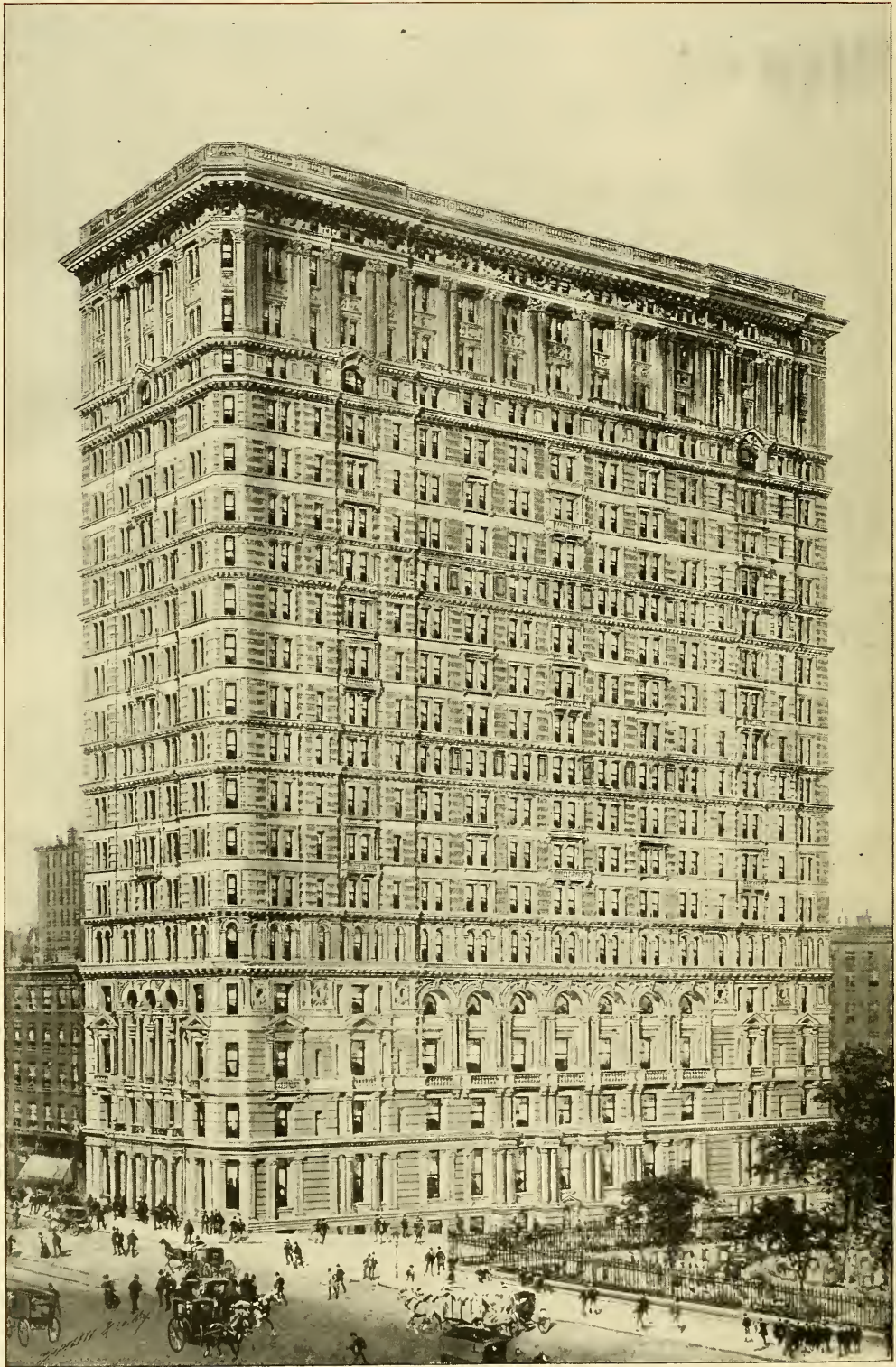
Empire Building, New York. 911 H.P. Babcock & Wilcox Boilers.
